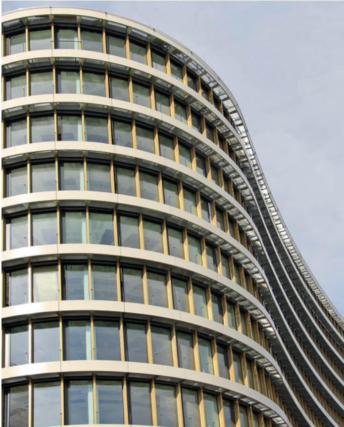
ENTERPRISE OFFICE CENTER – systém WICONA
